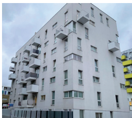
High-risk residential buildings
