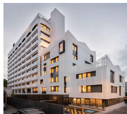
Purpose-built student accommodation
